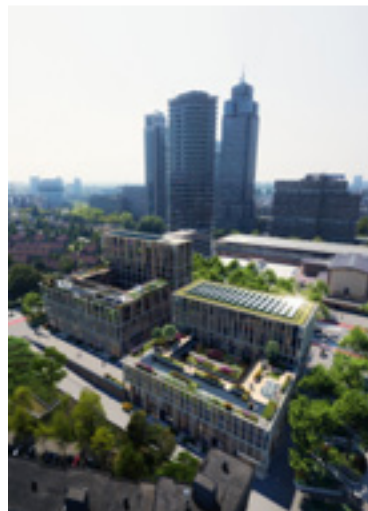
Above: Blocks B&C, mixed-use project in Amsterdam with nature-inclusive design combined with climate adaptive design features. Expected realization 2022.
