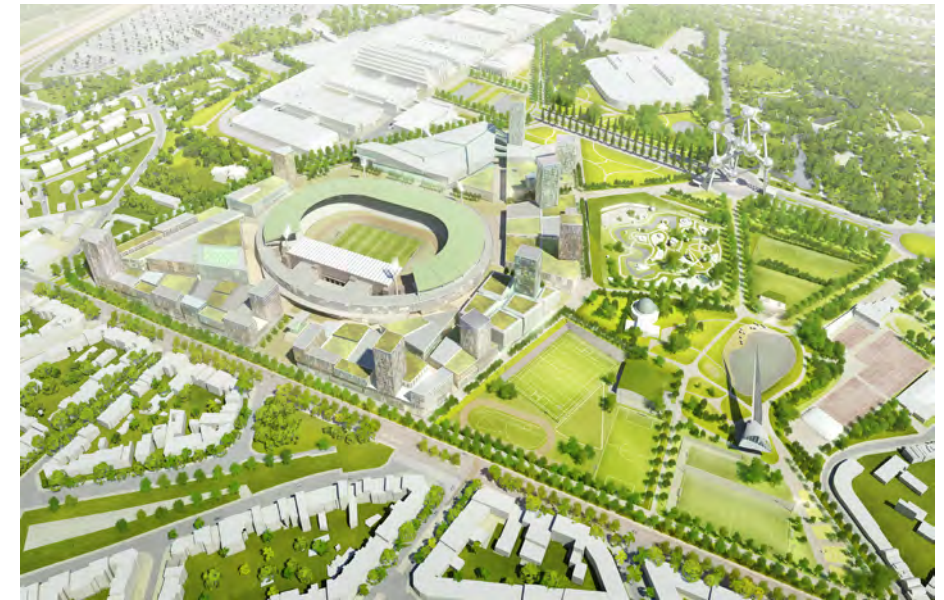
Redevelopment of 68 acre Heizel area in Brussels (former 1958 world expo area). Addition of more than 600.000 m 2 of real estate including the largest shopping center and the largest convention center of Belgium, 750 apartments, 7.000 build parking spaces and a new national football stadium. Fakton does the feasibility studies for the project and advises on the investment-, tendering-, phasing and parking strategy.
